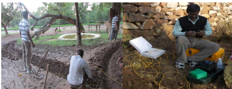
Fiber Optic Sensor Cable Deployment at Chhatbir Zoo & Panna
